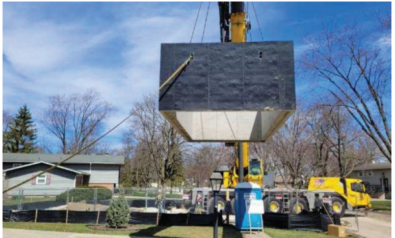
New precast concrete valve vault being set at the Centex Lift Station. See more about the Centex Lift Station Replacement below.
