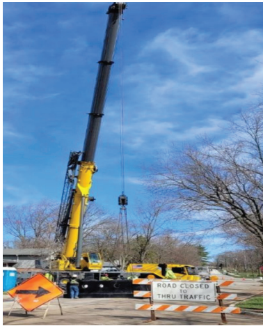
New precast concrete valve vault being set at the Centex Lift Station. See more about the Centex Lift Station Replacement below.
