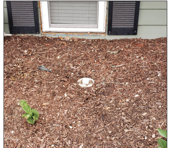
Example of a cleanout being installed (top) and a finished installation (bottom).
