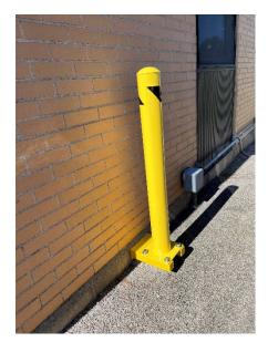
adjacent to a section of employee parking. Because the box couldn't be easily relocated and a standard bollard could not be mounted to the asphalt, Bill Smith fabricated a custom yellow bollard to protect the electrical box.
