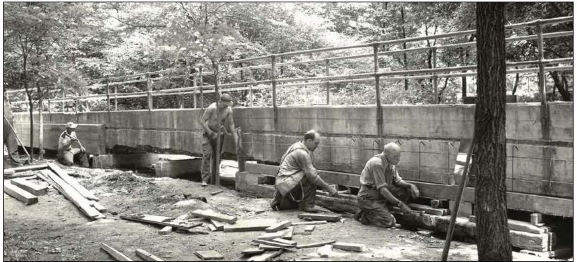
Historical photo of Maple Grove bridge being repaired.
