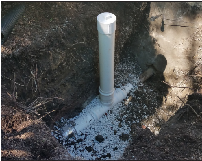
Example of a cleanout being installed.
