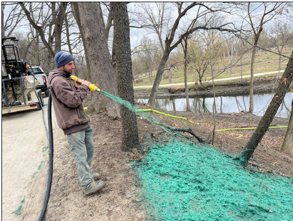
Plate 2. Photograph of the Hydroseeding of the Steep Slope at Fullersburg Woods (April 15, 2025)
