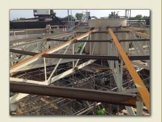
The recent Elmhurst digester cover replacement project is a great example of the successful application of Design-Build approach to construct needed emergency repairs quickly after the digester cover failed. Our Baxter & Woodman/Boller team was able to design and complete the improvements in a matter of months.
