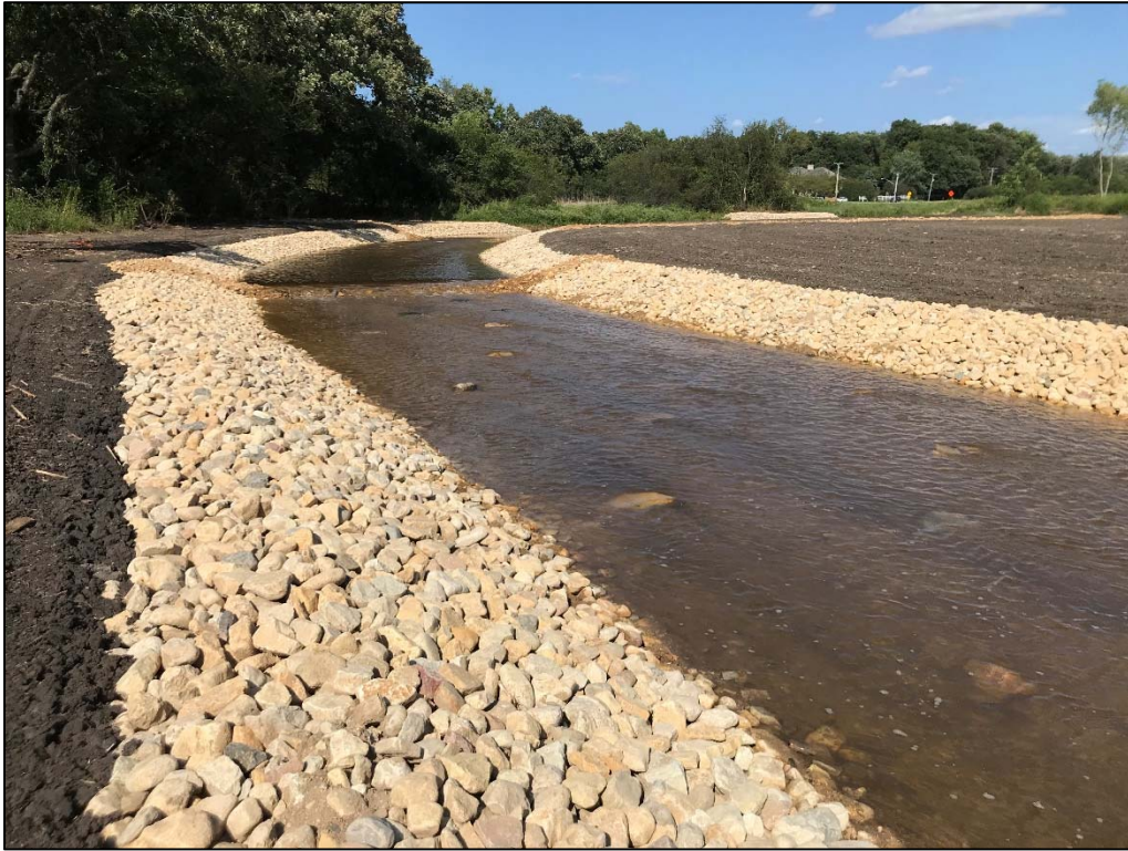
Plate 5. Flow of Spring Brook No. 1 was diverted into a new channel on August 27, 2020.
