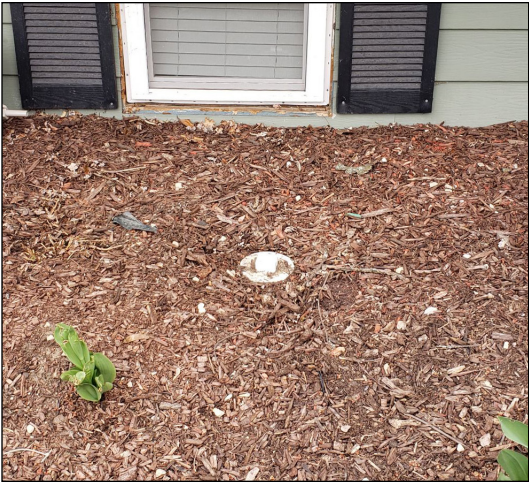
Example of a cleanout being installed (top) and a finished installation (bottom).
