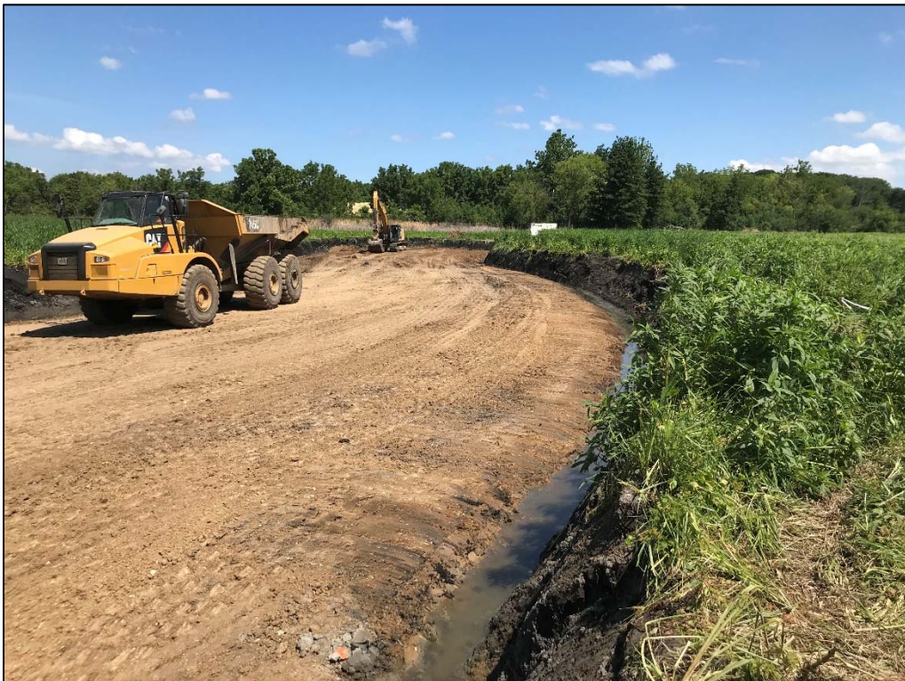
Plate 4. Excavation of a new Spring Brook channel in Reach B, a former impoundment created by a dam, continued in July 2020.
