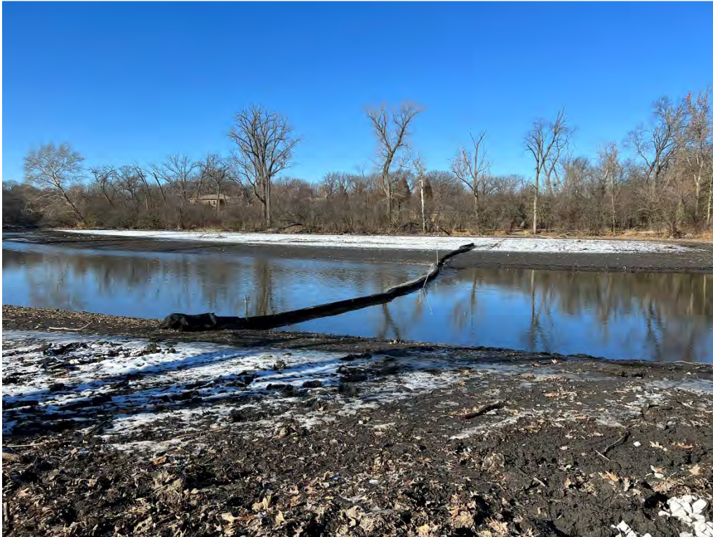
Plate 5. Photograph of one of the silt curtains utilized in the instream work (November 27, 2023).
