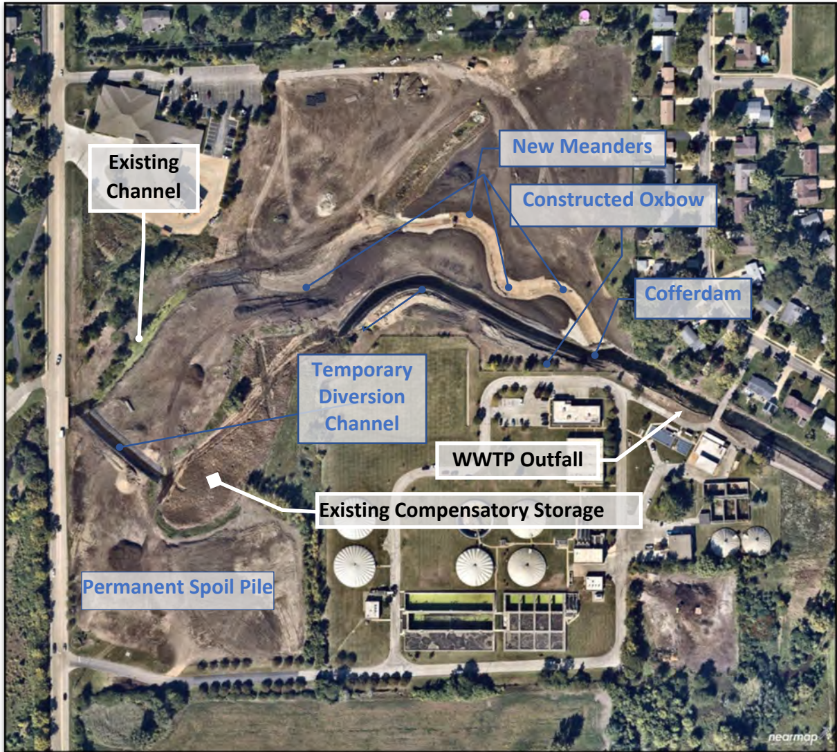
Plate 19. Aerial photograph of Klein Creek Streambank Stabilization Project (October 2022) By mid-October 2022 approximately \frac{2}{3} of the new channel had been excavated, with about \frac{1}{2} having also been filled with the new streambed material. Construction proceeded from upstream to downstream (east-to-west; right-to-left). The temporary diversion channel is to the south and partially cuts through an existing compensatory storage basin to save costs.
