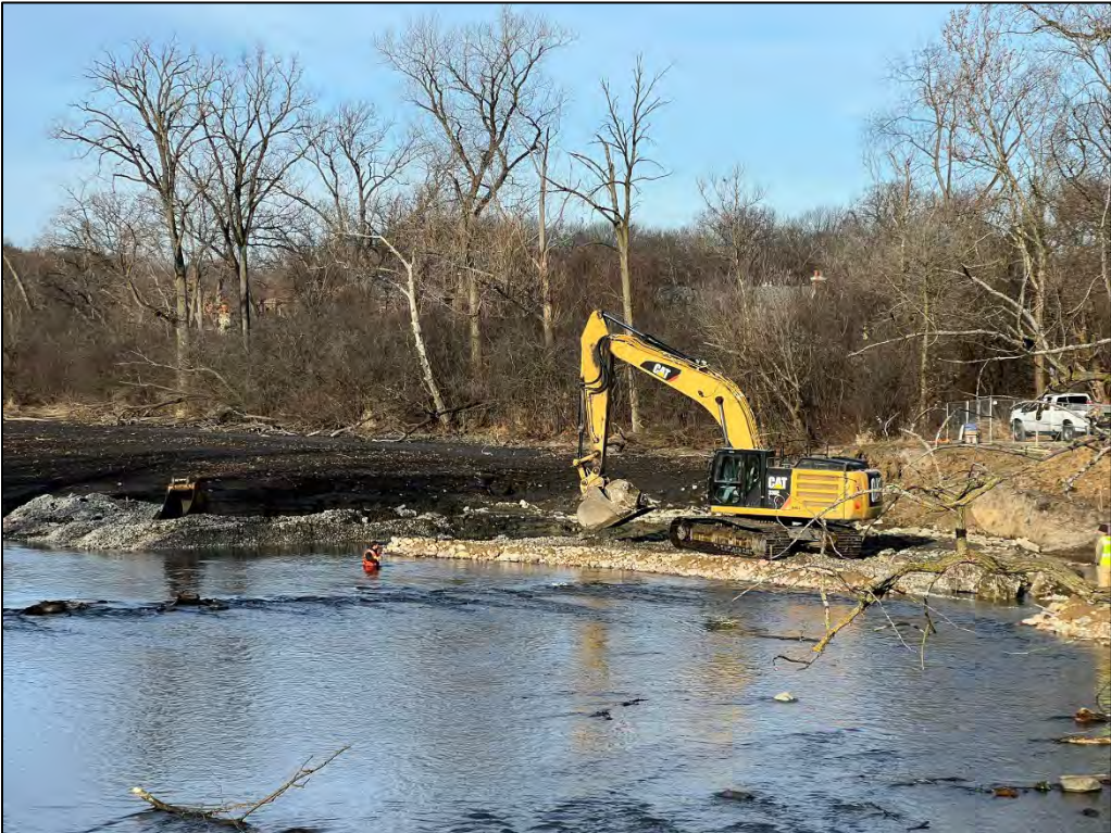
Plate 12. Photograph of the installation of a boulder in Riffle #1 (December 15, 2023)
