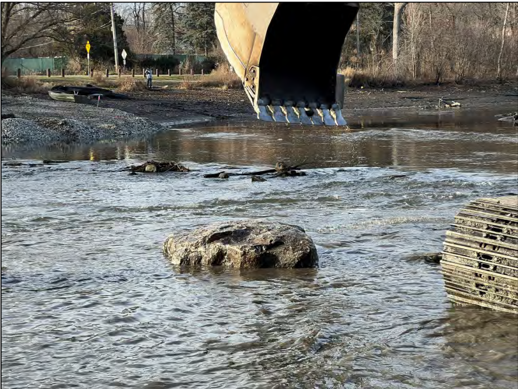
Plate 12. Photograph of the installation of a boulder in Riffle #1 (December 15, 2023)
