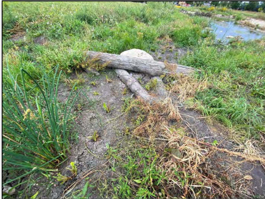
Plate 31. Looking downstream at a constructed oxbow in the previous streambed location. Wood harvested onsite and stabilized in place with boulders. Plugs are visible in the foreground during abnormally low flow conditions.
