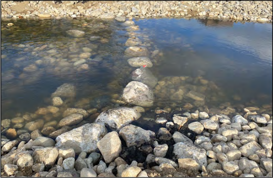
Plate 26. Photograph of a rock substrate area at the Klein Creek Streambank Stabilization Project. The rock substrate areas were designed to mimic a rock riffle by placing a weir of large boulders followed by a downstream stretch (photo left) of cobbled substrate. Due to the flat gradient, this boulder weir was installed “in-the-wet” to ensure that their tops were above the normal water level.
