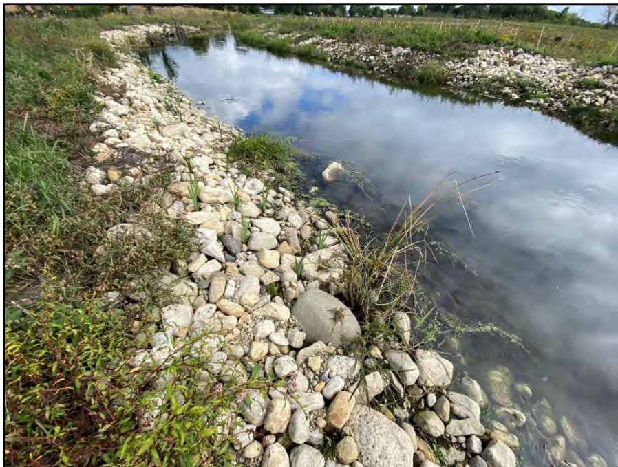
Plate 32. Looking downstream at the recently planted plugs within the vegetated rock toe.
