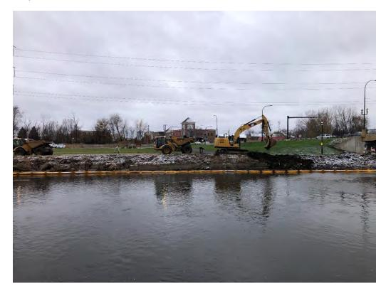
Plate 19. Photograph of the boulder toe installed on the west bank of the DuPage River (Winter 2025)
