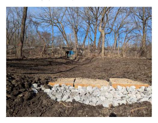
**Plate 32.** Photograph of Swale 5 after being seeded and stabilized with erosion control blanket (Winter 2025)
