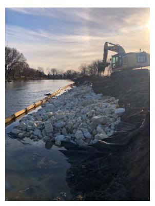
**Plate 20.** Photograph of the completed boulder toe with seed and erosion control blanket on the west side of the Lower DuPage River (Winter 2025)
