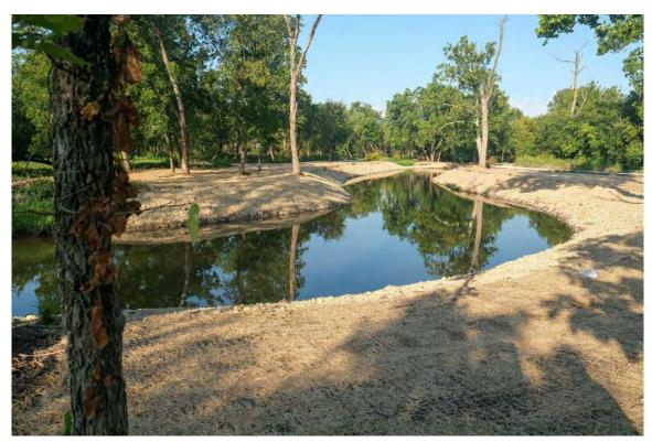
Approximately 1,000 linear feet of bank stabilization was also installed in Summer 2024. Due to field conditions observed post dam removal, some of the planned locations of streambank stabilization were relocated to areas with more severe bank erosion. Areas where bank stabilization was installed will be planted with perennial plugs in Summer 2025. Plate 10 is a photograph of a section of streambank stabilization at Fullersburg Woods. Riffle 8 is also shown in the photograph.
