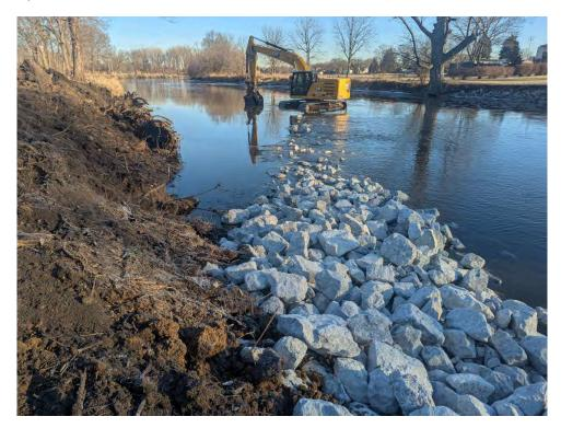
**Plate 25.** Photograph of a brush box being installed on the east side of the Lower DuPage River (Winter 2025)
