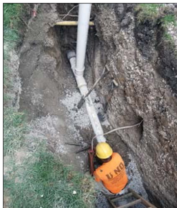
Examples of cleanouts being installed (left and middle) and a finished installation (right).
