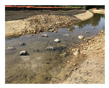
Section of Spring Brook Phase 2 channel under construction. Note the riffle in the foreground. Riffles, due to their flow patterns and structure, are biological hotspots.
