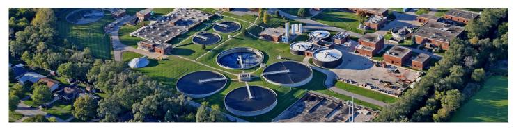
Aerial view of Glenbard Waste Water Treatment Plant, capable of treating an average of 16 million gallons of waste water a day before discharging to the East Branch DuPage River.
