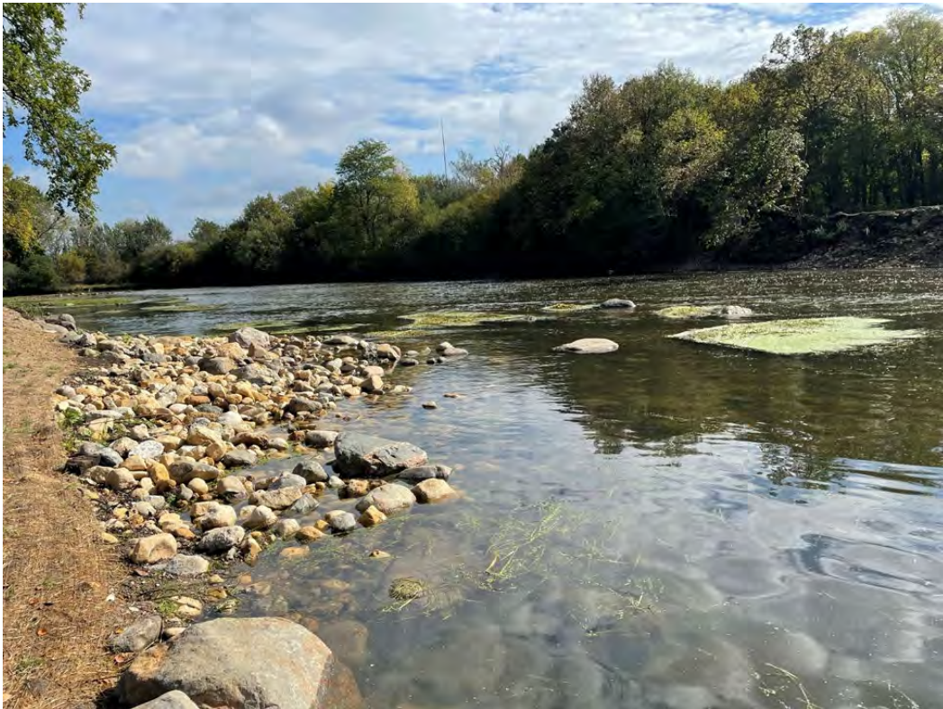
Plate 4. Free-flowing DuPage River, Looking Upstream; Toe Rock and Boulder Array along West Side
