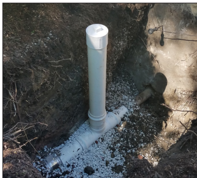
Example of a cleanout being installed (left) and a finished installation (right).
