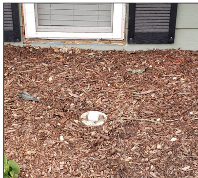
Example of a cleanout being installed (left) and a finished installation (right).
